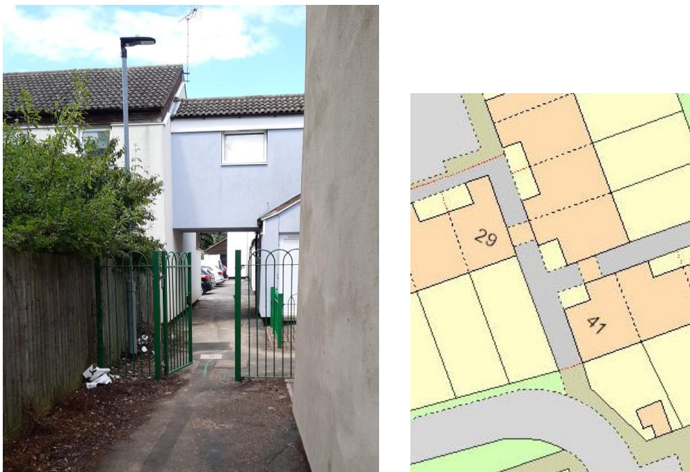
Highway adjacent 41 Crabtree Paston Photos July 2020 – gate insecure
