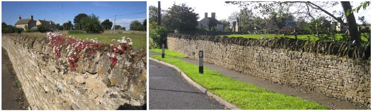
Stone boundary walls
