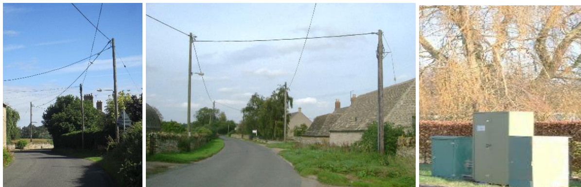
Posts and overhead utility wires
