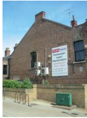
Western extent of Cowgate
